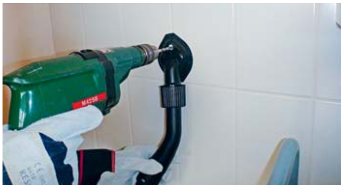
Loch in Platte bohren
